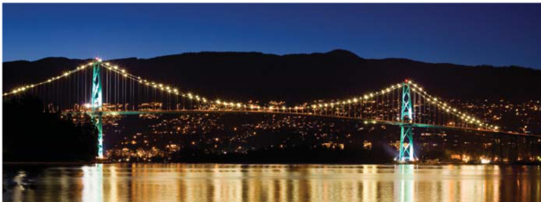
Lion's Gate Bridge, Vancouver
